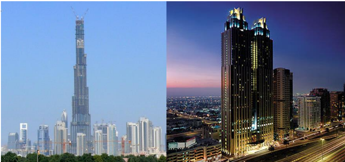
Figura 2-4 – a) Burj Dubai Tower; b) Shangri-La Hotel.
