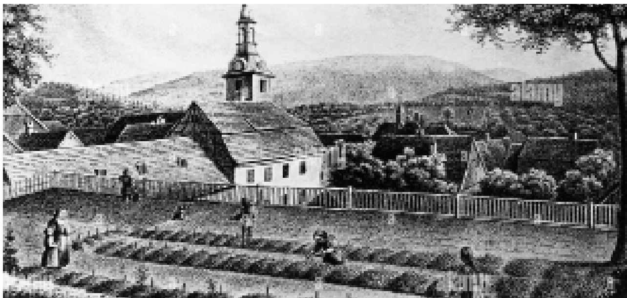
Fig.1 - Kindergarten of Friedrich Froebel in Bad Blankenburg
