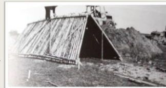
Construction of Observatory, 1971, Robert Morris.
