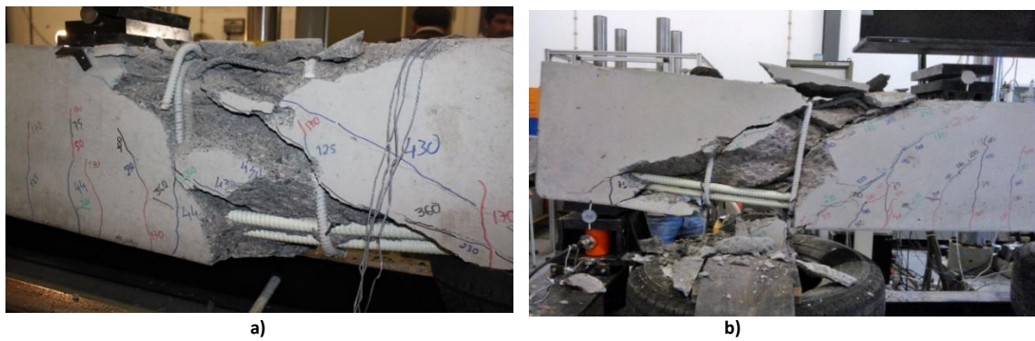
Figure 80 – Shear failure due to the crushing of the concrete rod: a) BS250GFRP2; b) BC250GFRP2
