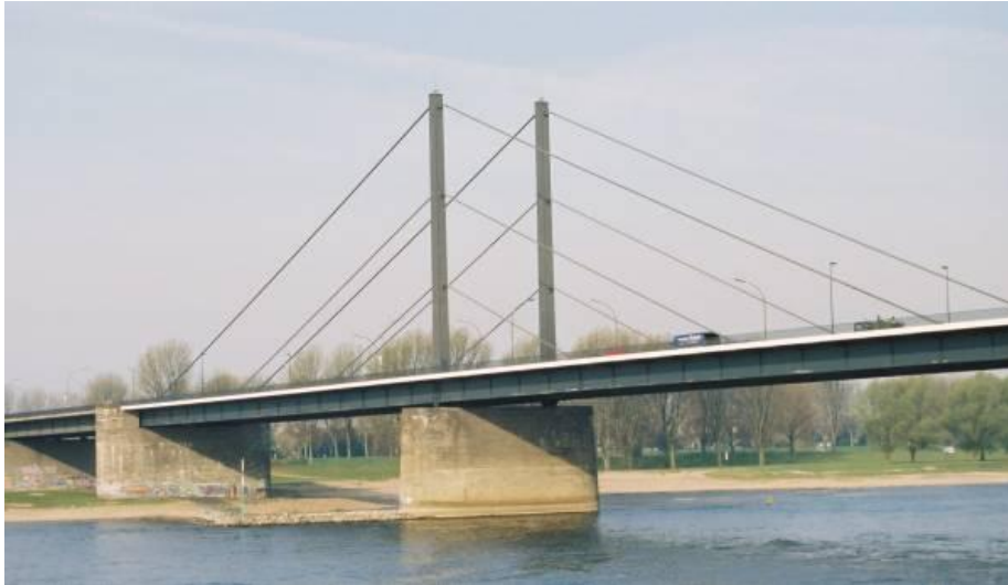
Figura 19 Ponte Theodor Heuss [1]
