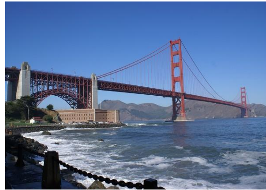
Figura 18 Ponte Golden Gate [1]
