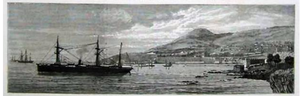
6. The (...) lane end of the Brazilian Submarine cable at Madeira.
