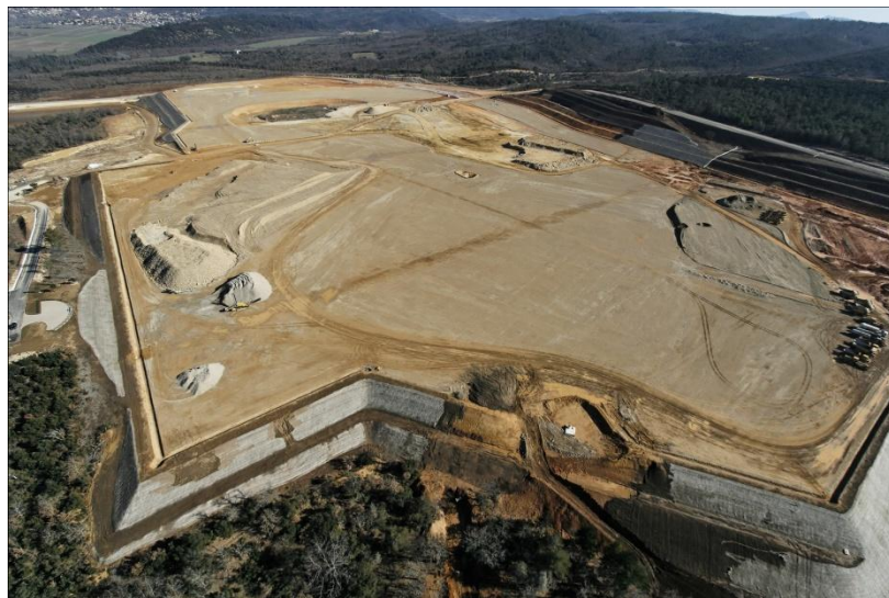
Figure I-1: Aerial view of the ITER construction site
