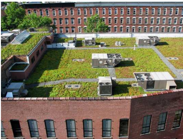
Picture 4.8: Green Roof of the Garden Street Lofts in Hoboken, New Jersey Source: ne-rest.com (06/08/2010)
