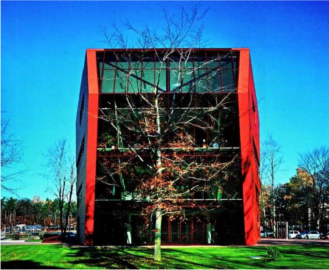
Picture 5.3: South façade Source: Celik, M. (2007)
