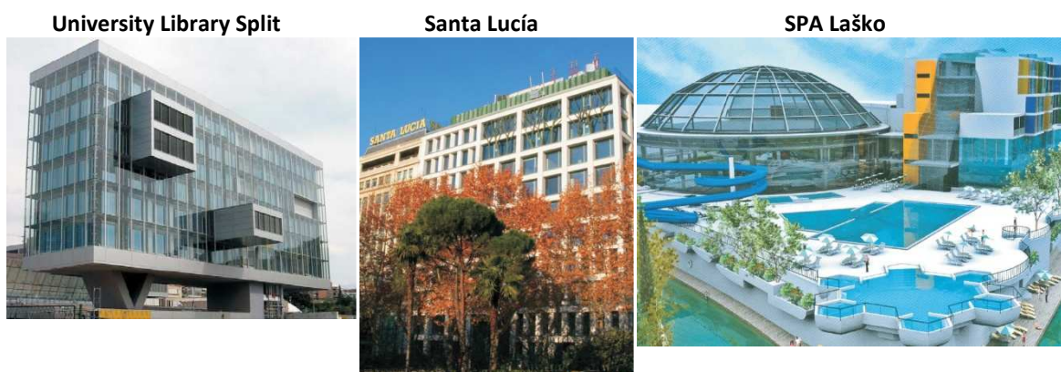
Picture 5.10: Intelligent buildings Source: Menerga d.o.o.
