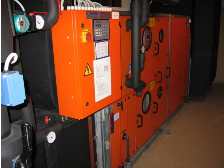
Picture 5.7: Air-conditioning unit with high efficient regenerative heat recovery Source: Celik, M. (2007)
