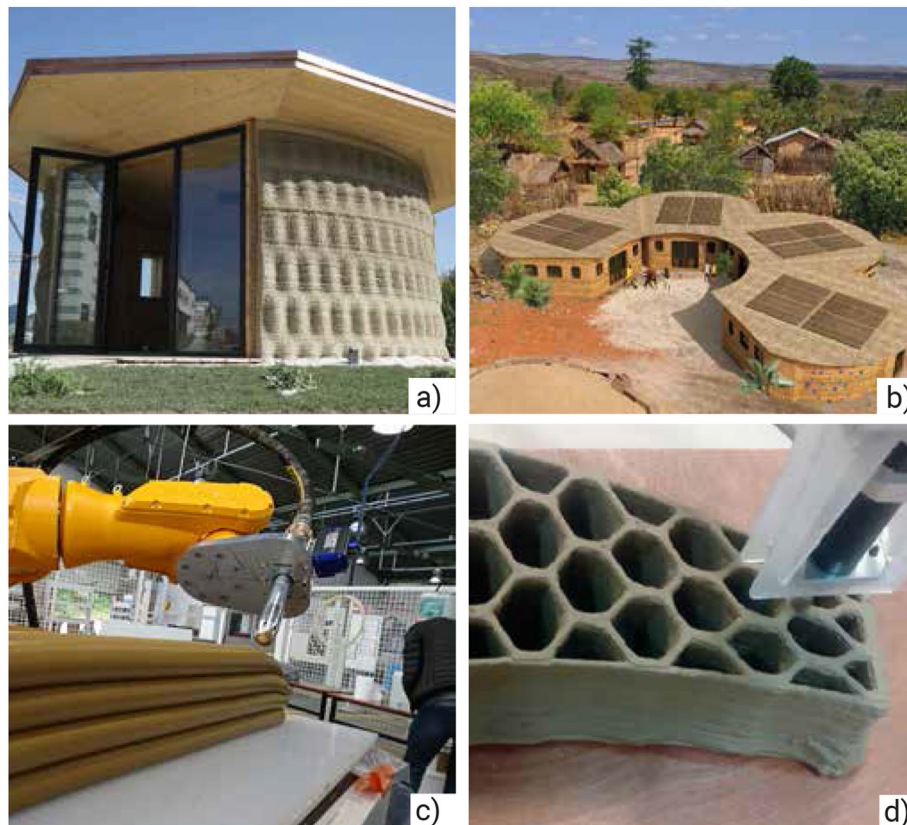
Fig. 11 Structures printed using clay or soil-based materials: a) 3DP house "Gaia" printed by Wasp using soil-based materials (WASP, 2018); b) Project for a future 3D printed school by Studio Mortazavi; c) Printing process using a circular nozzle and a soil-based material developed by Perrot, Rangeard and Courteille (Perrot et al., 2018); and d) Structure printed by Kontovourkis and Tryfonos (Kontovourkis and Tryfonos, 2020a), using an extruder developed by 3D Potter.
