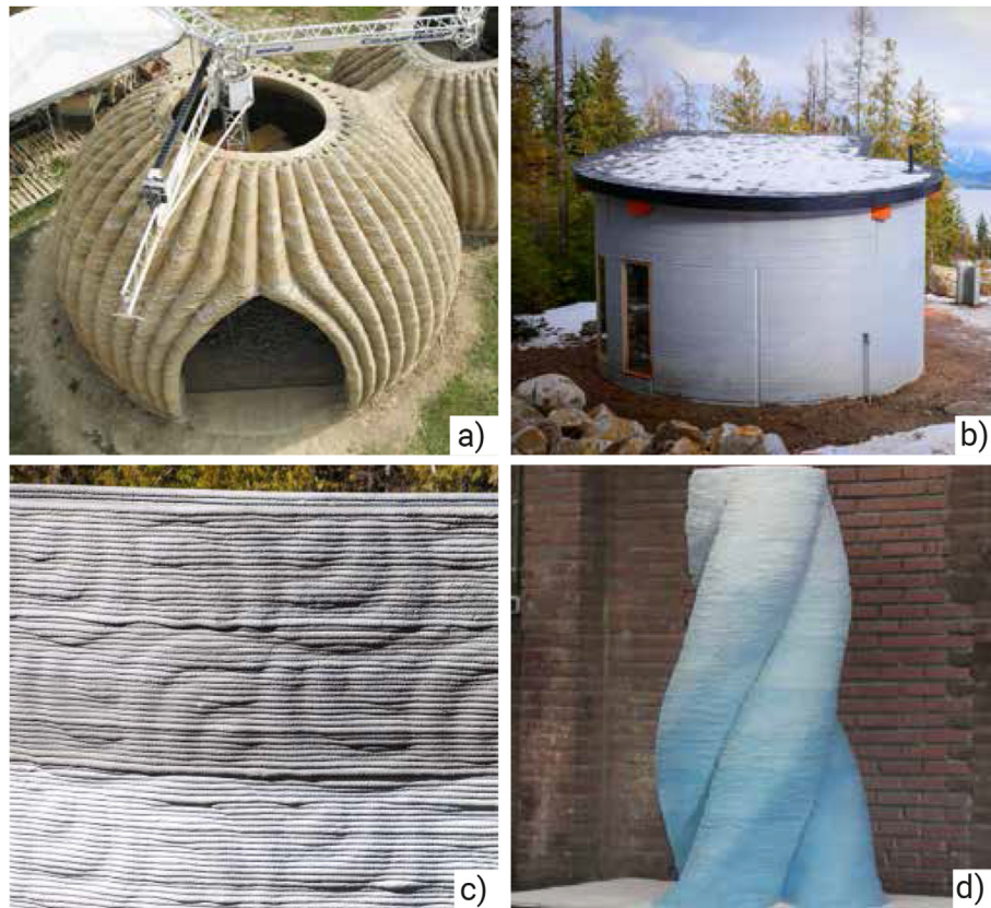
Fig. 1 Structures printed with different materials and technologies: a) “Tecla” printed with soil by WASP and designed by MC A – Mario Cucinella Architects (WASP, 2021b); b) and c) Structures printed by TAM, using 3DP to explore new textures and geometries (Twente Additive Manufacturing B.V., 2021); and d) colour gradient mortar explored by Bruil, in the Material Xperience exhibition in Rotterdam (Bruil, 2021; Bruil and MaterialDistrict, 2016).
