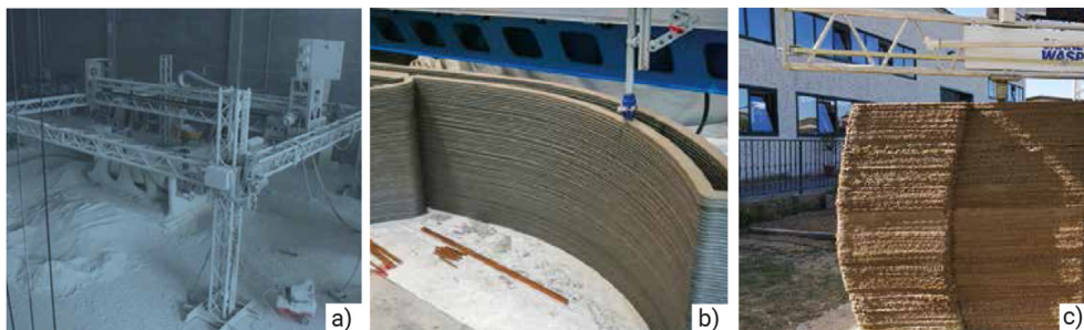
Fig. 3 3DP process types used in construction: a) D-Shape technology, BJ method (D-Shape, 2010); b) ME method, robotic arm printer by TAM (Twente Additive Manufacturing B.V., 2021); and c) ME method, Crane printer by Wasp.
