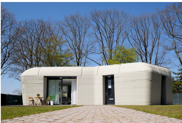
Fig. 5 3D printed house project designed by Houben & Van Mierlo Architecten for Project Milestone (2018).
