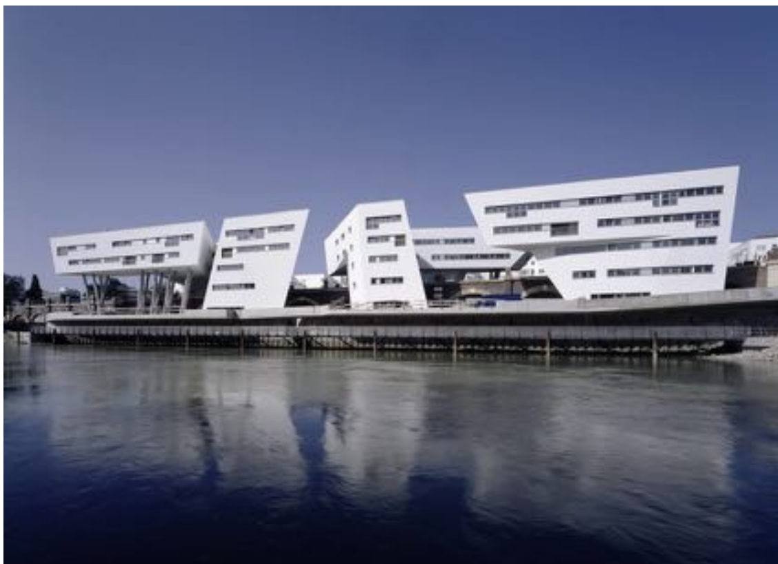
Figura 15: Spittelau Viaducts Housing Project.
