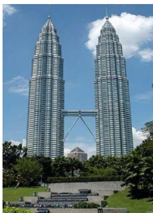
Figura 17. Petronas Twin Towers, Kuala Lumpur, 1996 (Rosa, 2011)
