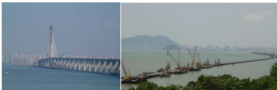
Figura 2.4 - Shenzen Western Corridor, Hong Kong [16,25]
